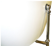
Non-pedestal drain kit installed above floor.
